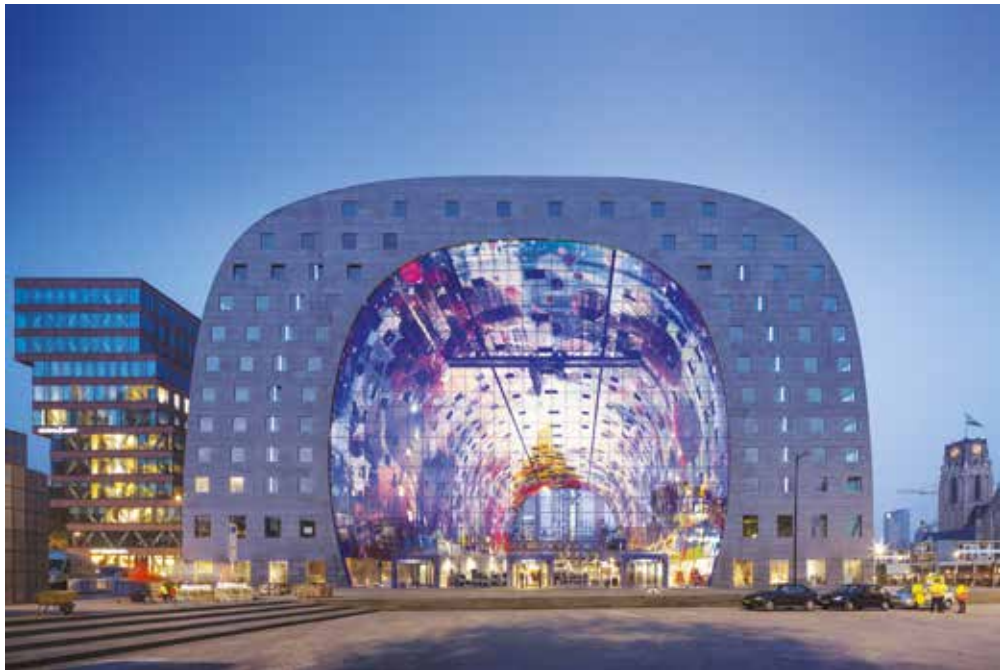
Markthal, MVRDV, Rotterdam, Paesi Bassi/The Netherlands, 2014, Foto/Photo Daria Scagliola & Stijn Brakkee
